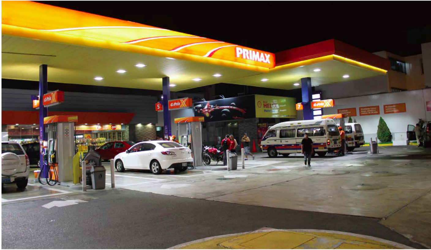
Primax Petrol Station, Peru
