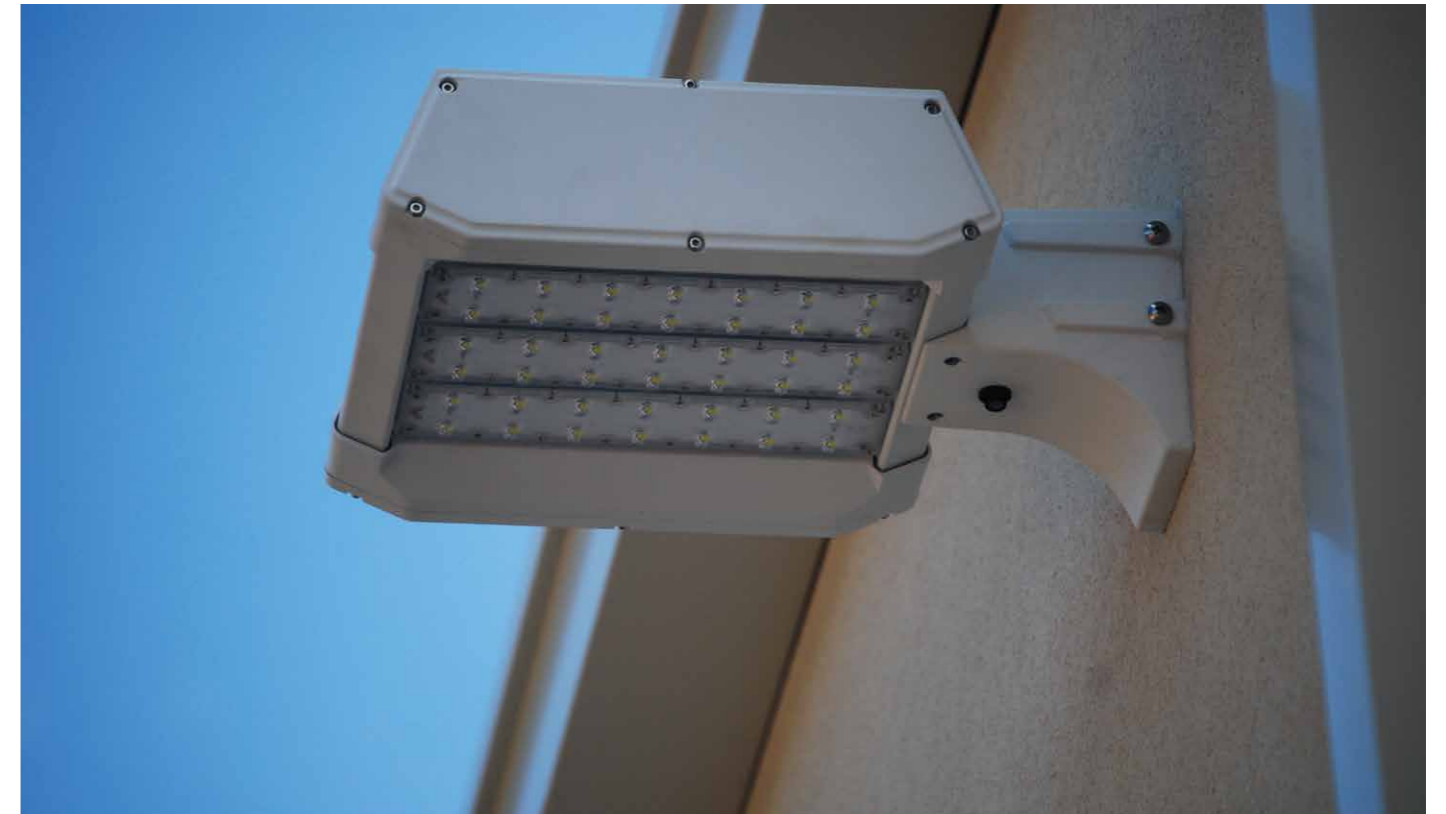
Richifield Building G.A. USA
