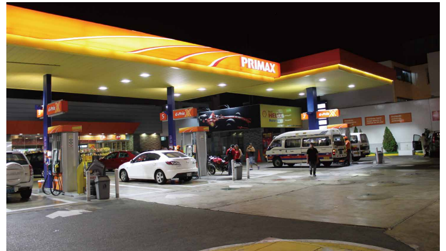
Primax Petrol Station, Peru
